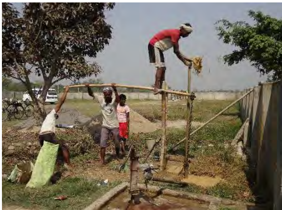
5. Digging wells by manual (Photo: March 2012)
