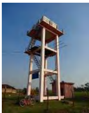
Photo 5.1 Water Tower for Waterworks (Goini)
