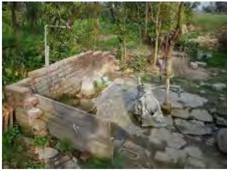
Photo 5.3 Waterworks drawn through pipes from subsoil water at the foot of the mountain (Suryapura)
