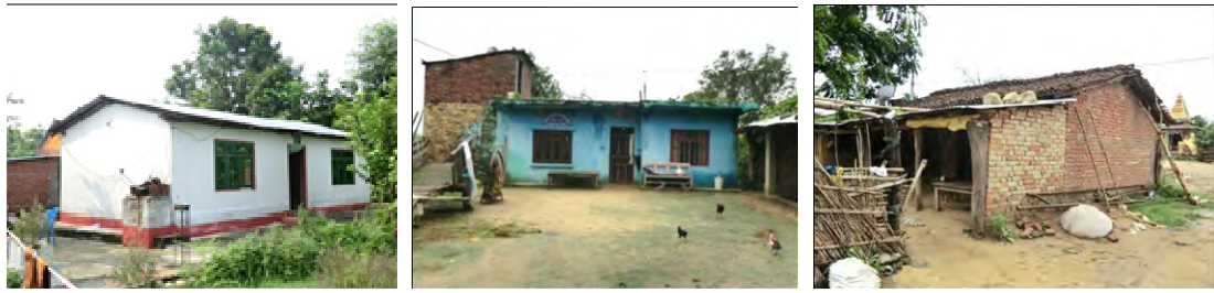
Zinc-coated steel roof
